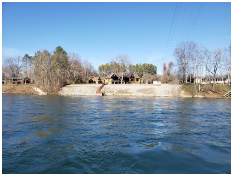
Land Owner has added rock riprap to slow erosion after riparian area was cleared.
