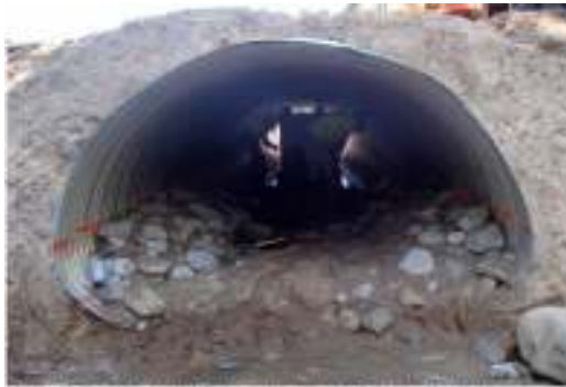
Photo 4. Placement of stream bottom material inside of pipe arch, looking upstream.
