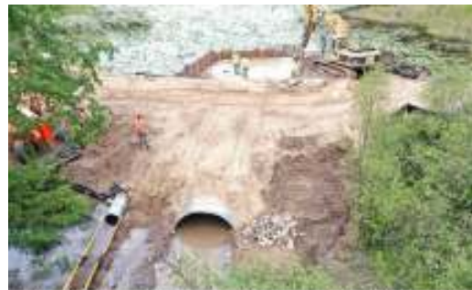
Photo 6. Propping for short pile removal, note the downstream structure at left of pipe arch outlet.
