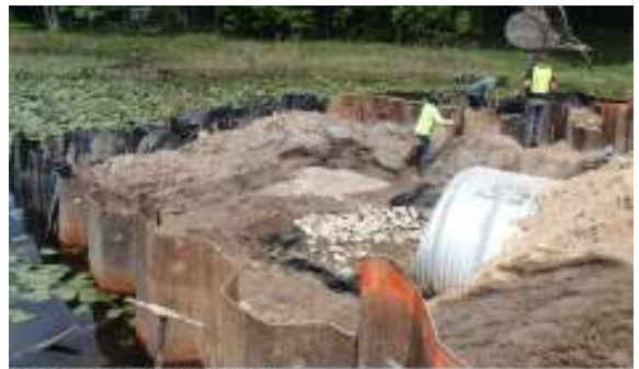
Photo 5. Propping raft for short pile removal.
