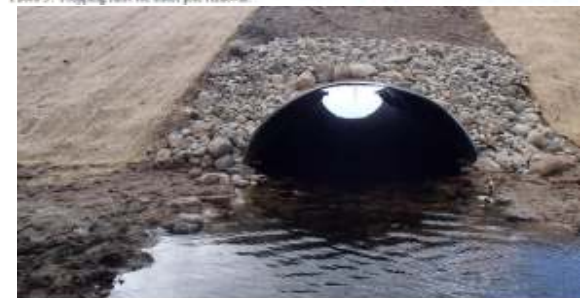
Photo 7. Upstream view of pipe arch.
